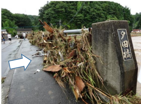
(a) Driftwood accumulations around the Yuuta Bridge.
