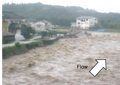
(b) Left bank of 5.8km point.
