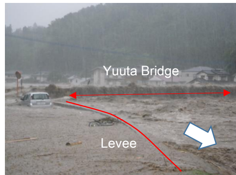
(b) Overbank flows around the Yuuta Bridge.
