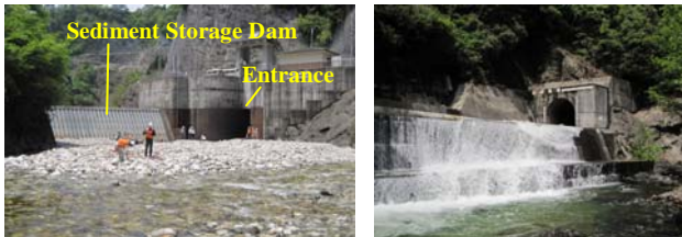
Figure 2. (Left) Entrance Viewed from Upstream (Right) Exit of Bypass Tunnel
